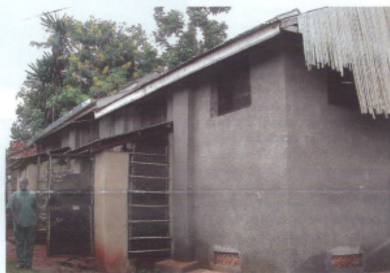
Brick built growing rooms. The doors filled with wet charcoal help with humidity.
