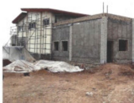
Lab under construction at Mohammed Entessari's new compost plant.
